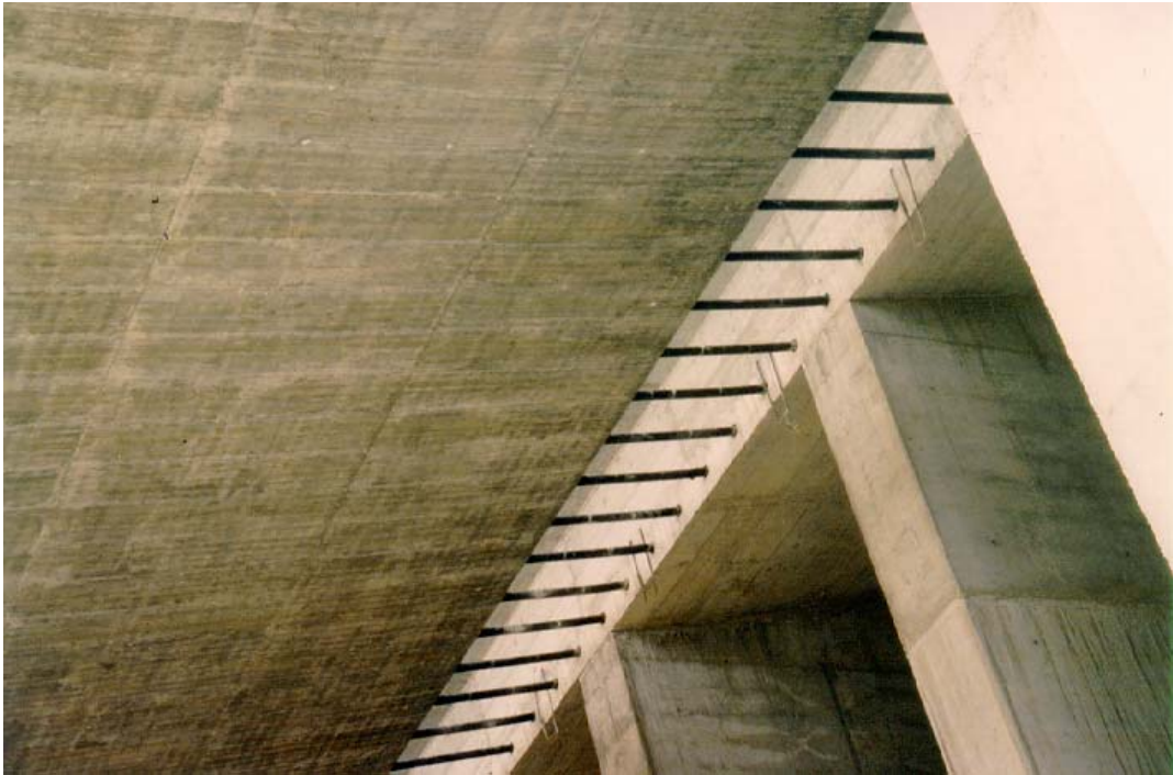
Figure 5 - Detail of Canopy, Cables and Fins
