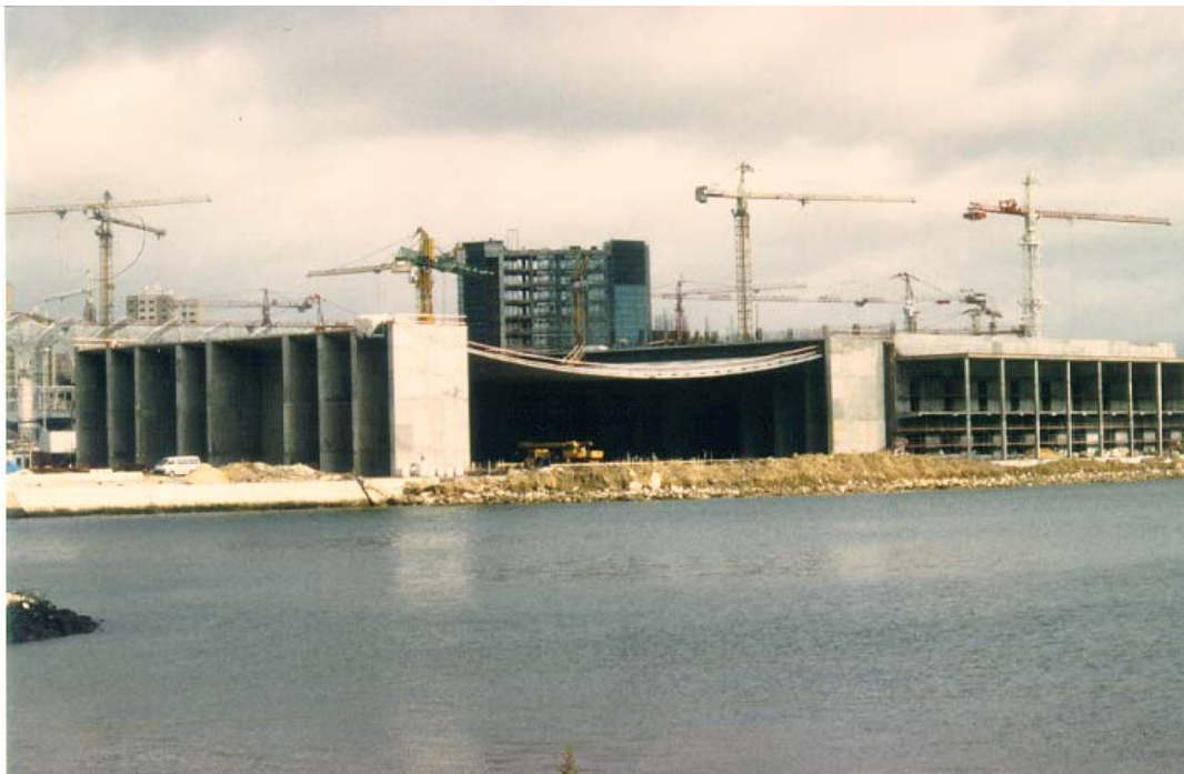
Figure 6 - General View of Canopy
